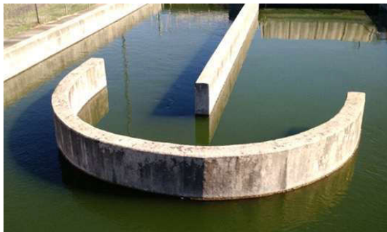
Figure 7b: Part of Aerator (Aeration Basin).
