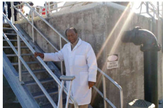
Figure 6a: Inlet pipe to Wastewater treatment plant.
